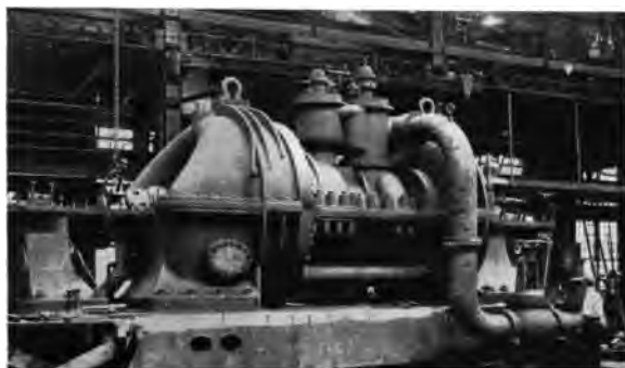
Erecting 7,500 HP Steam Turbine
